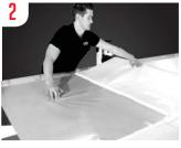
Lower roller onto media and substrate. Separate liner over the top of the roller.
