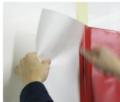
4. Hold the edge of the graphic smooth and taut away from the application surface with one hand and squeegee horizontally from the centre towards the outer edges. The first squeegee stroke should be next to the hinge where the adhesive has been exposed. Continue squeegeeing, using firm overlapping strokes from the centre out, working away from the starting point. .
