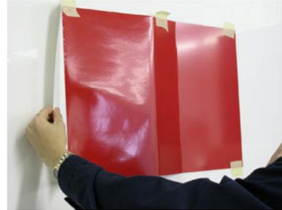
4. Re-squeegee the entire graphic using very firm squeegee pressure, including all edges. Puncture any air bubbles with a straight pin and re-squeegee from the edge of the bubble towards the puncture.
