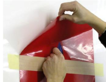
5. Once the upper portion is applied remove the hinge so that the lower portion of the graphic can be applied.
