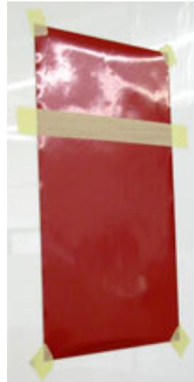
3. Separate the upper portion of the liner from the graphic and remove this section of the liner by cutting it with a scissors or razor knife. Use the knife at an angle to make avoid cutting into the wall surface or the graphic.
