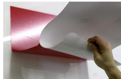
7. Hold the bottom edge of the graphic smooth and taut, away from the application surface with one hand and squeegee horizontally from the centre towards the outer edges. Continue squeegeeing, using firm overlapping strokes from the centre out, working away from the starting point. Pull the liner back as necessary.
