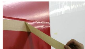
6. Reach behind the graphic and carefully pull the liner back several inches to expose the adhesive.
