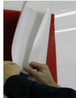
7. Hold the bottom edge of the graphic smooth and taut, away from the application surface with one hand and squeegee horizontally from the centre towards the outer edges. Continue squeegeeing, using firm overlapping strokes from the centre out, working away from the starting point. Pull the liner back as necessary.
