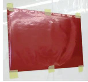
2. Reach behind the graphic and carefully pull the liner back several inches to expose the adhesive.
