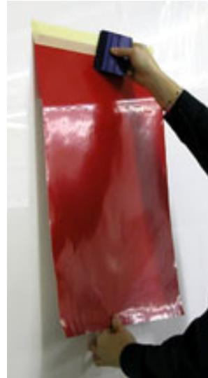
5. Re-squeegee the entire graphic using very firm squeegee pressure, including all edges. Puncture any air bubbles with a straight pin and re-squeegee from the edge of the bubble towards the puncture.
